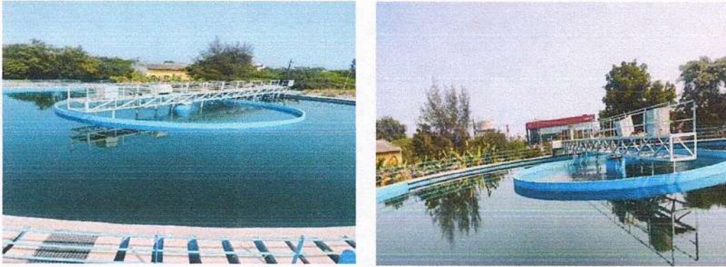
Fig. Clarifocculator.
