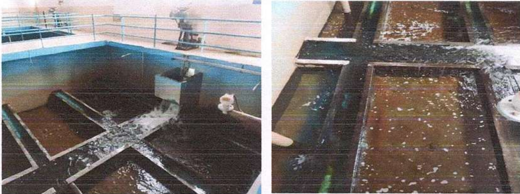
Fig. Rapid Sand Filtration Bed.
